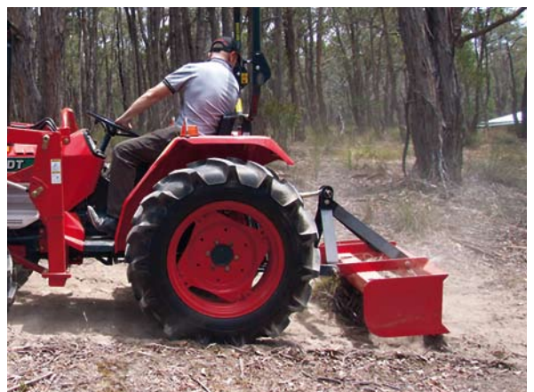
Grading - Tines up - Spreading soil while collecting debris
